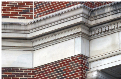
A cornice constructed of limestone may have vertical joints offset from course to course.
