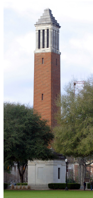
Towers, such as Denny Chimes, taper as they rise. The tower’s “heavy” base withstands the weight of the shaft.
