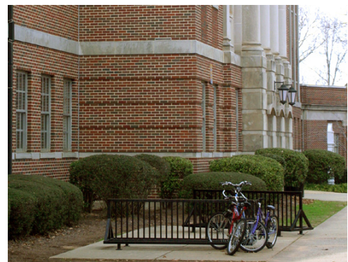
Brick bases, as shown in these images can lend the appearance of rustication, as with stone bases.
