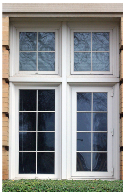
Above: Historic example of the stacked window design
