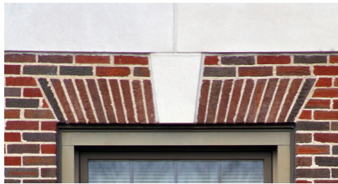
Example of a flat or jack arch used on campus.
