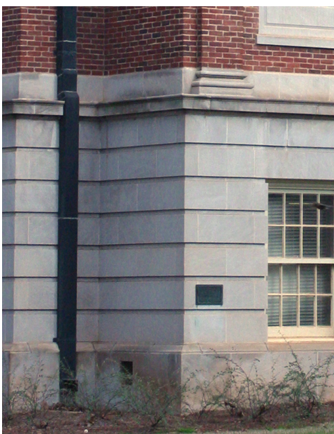
Above: Base projecting outward from the shaft.
